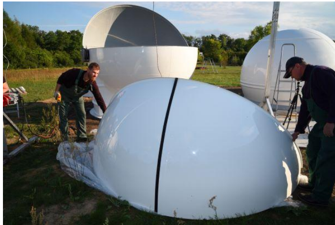
Figure. 44 – Orientation and preparation of Shutter No. 2 for installation
