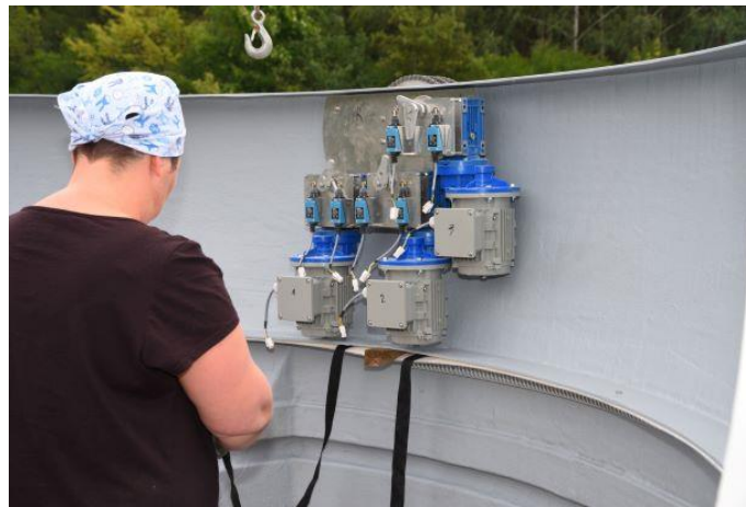
Figure. 6 – putting the transport slings between the top and bottom part of the observatory base
