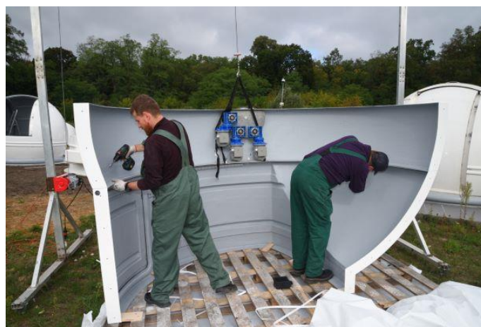
Figure. 7 – dismantling of M6 screws connecting the top and bottom of the observatory base to be transported to the installation site
