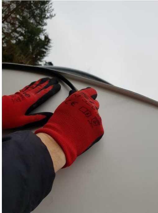
Figure. 68 – mounting the seal on edge of shutter #2
