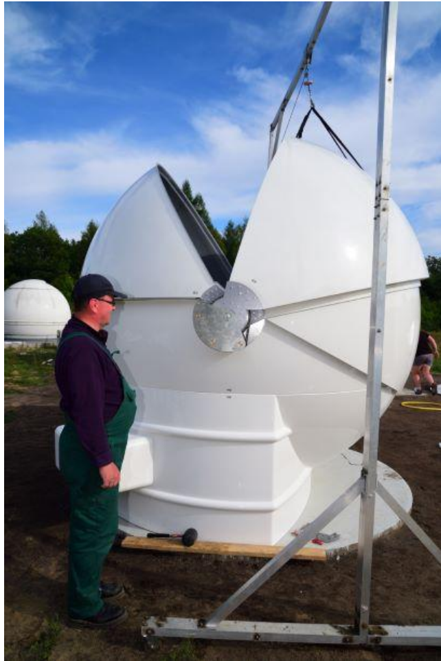
Figure. 54 – mounted shutter No. 3 mounting in its handles
