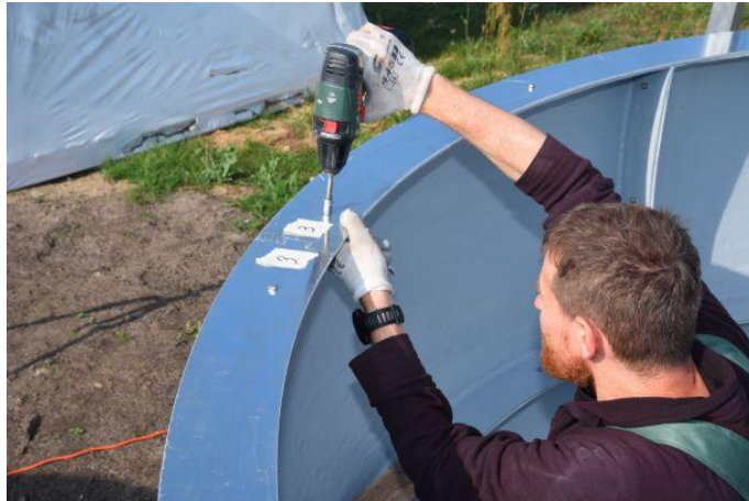
Figure. 31 – Connecting the stiffening ring from the base of the observatory
