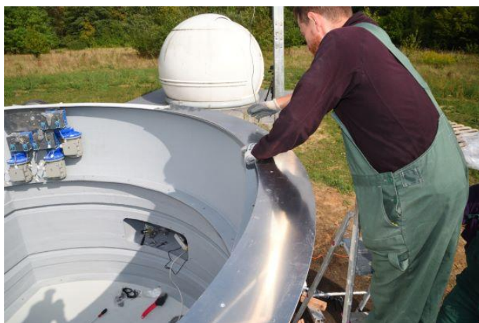
Figure. 29 – Securing the ring with mounting screws
