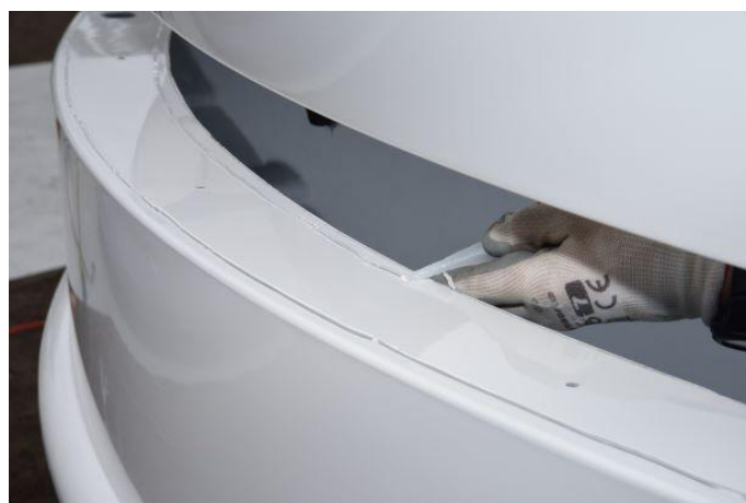
Figure. 21 – sealing of the observatory base elements
