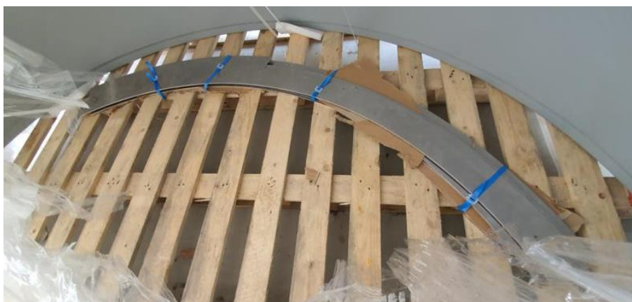
Figure. 3 – elements of the upper ring stiffening the base of the Clamshell observatory
