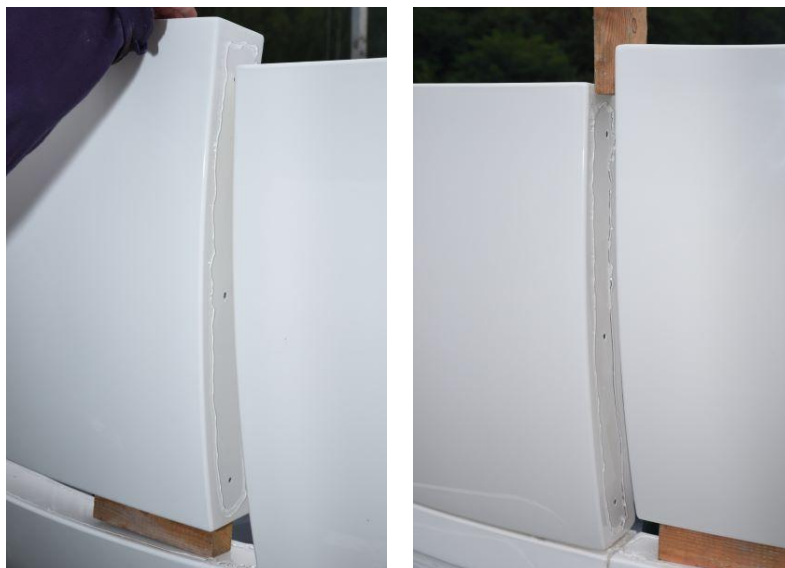
Figure. 23 – Place of sealing of the upper elements of the observatory base
