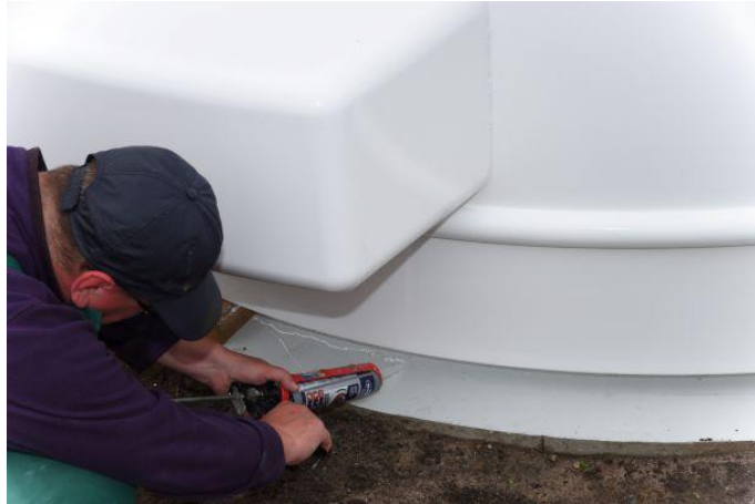
Figure. 14 – applying seals under the base of the observatory
