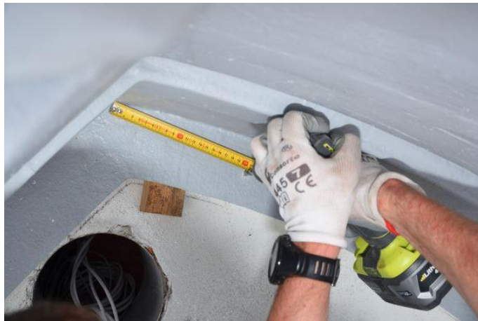
Figure. 12 – drilling of base fixing holes
