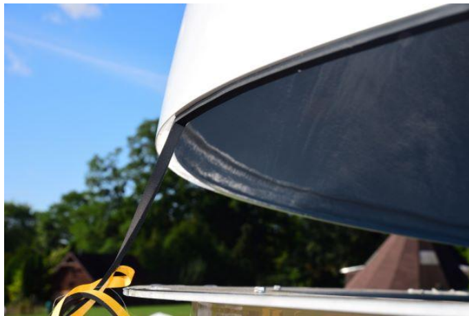
Figure. 65 – Installation of the gasket on the edge of shutter No. 1.
