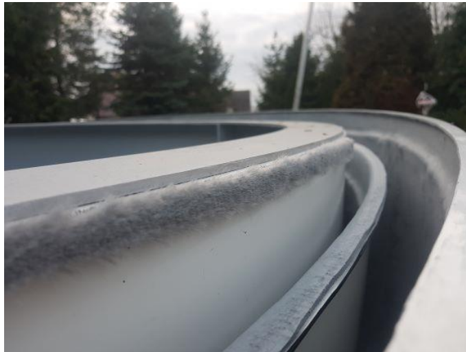
Figure. 71 – How to install the seal under the upper ring
