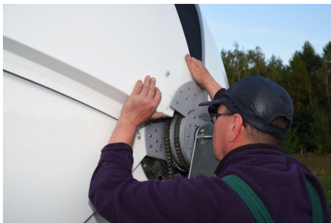
Figure. 53 - Shutter No. 3 mounting in the handles - left view
