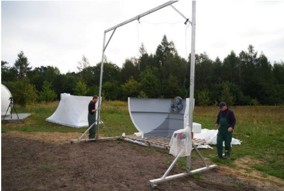
Figure. 4 – electric gantry used for observatory mounting
