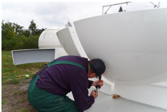
Figure. 16 – applying seals on the planes connecting the base
