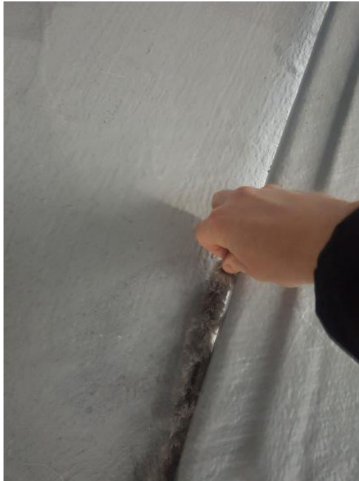
Figure. 70 – Installation of the gasket on cover 3
