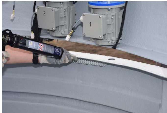
Figure. 20 – sealing of the observatory base elements
