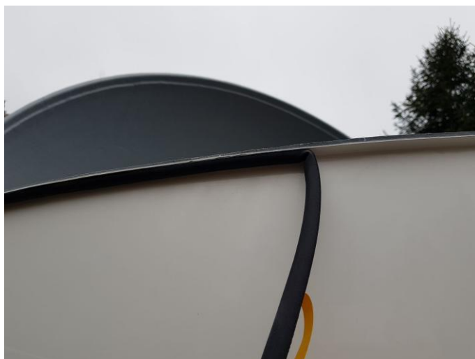
Figure. 67 – mounting the seal on shutter #2
