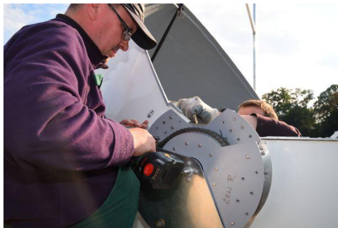
Figure. 42 – screwing the shutter #1 to its mounting handle
