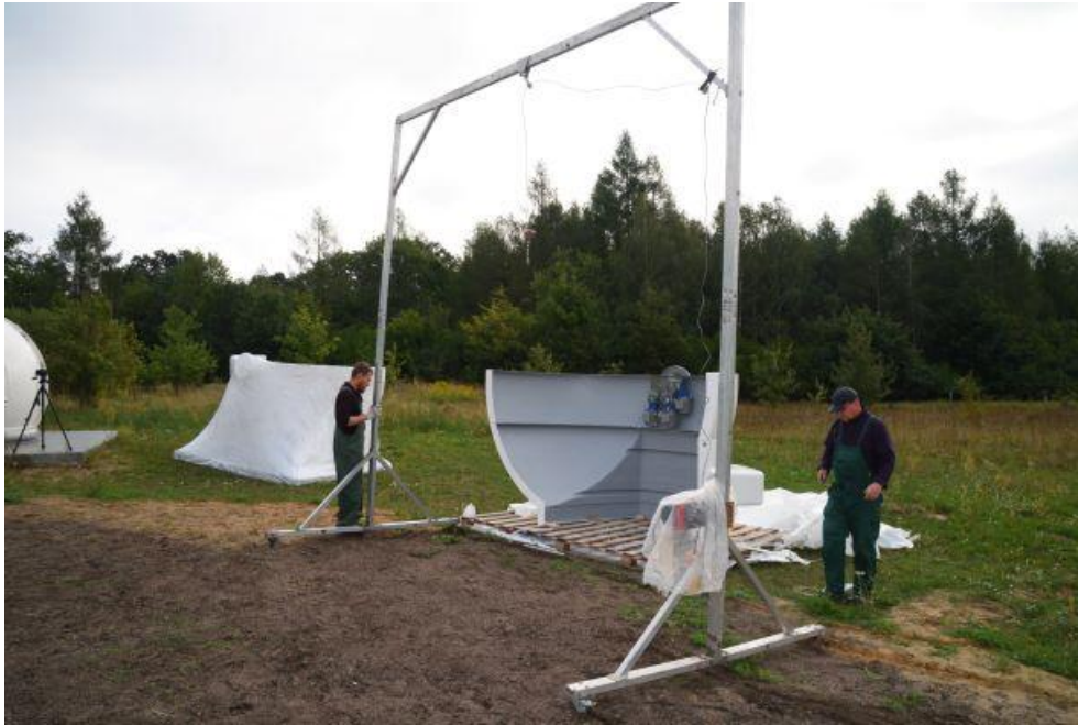
Figure. 4 – electric gantry used for observatory mounting
