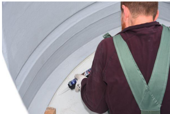
Figure. 15 – applying seals under the base of the observatory
