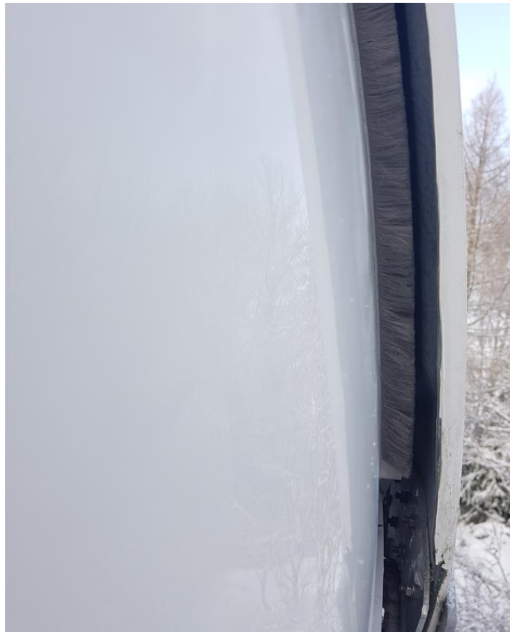
Figure. 70 – Placement of the seal on back edge of shutter #1
