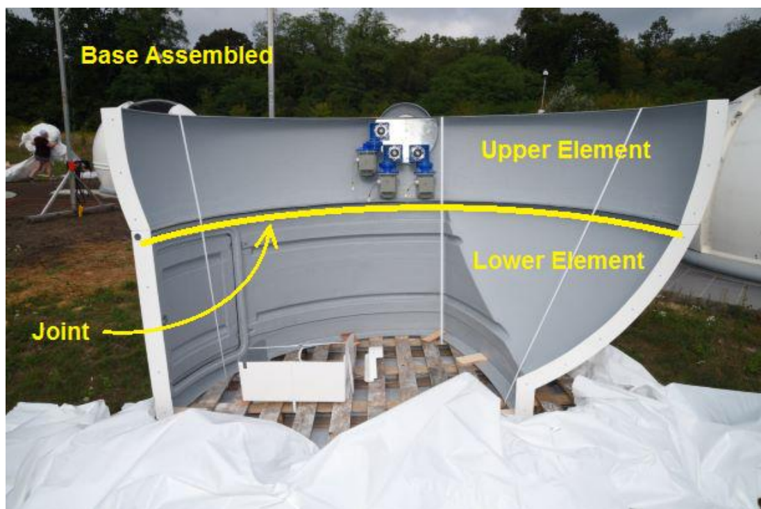
Figure. 5 – unpacked left part of the observatory base, with upper and lower segments defined
