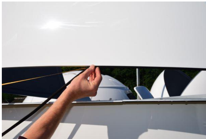
Figure. 64 – Installation of the seal on the edge of shutter No. 1.
