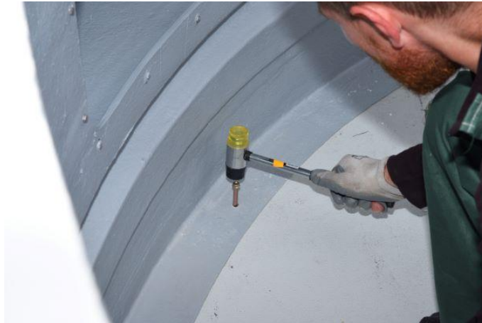
Figure. 17 – mounting the base with anchors
