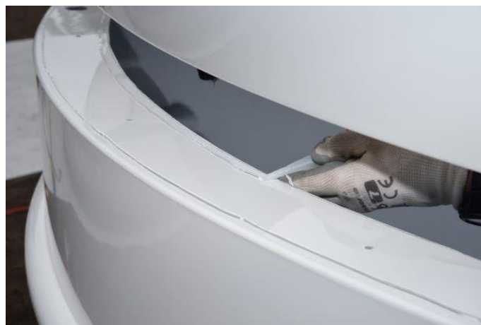
Figure. 21 – sealing of the observatory base elements
