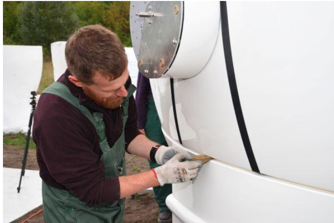
Figure. 22 – Lowering the upper base element onto lower one
