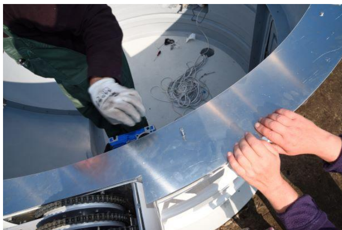
Figure. 30 – Mounting the side elements of the stiffening ring
