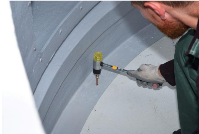
Figure. 17 – mounting the base with anchors
