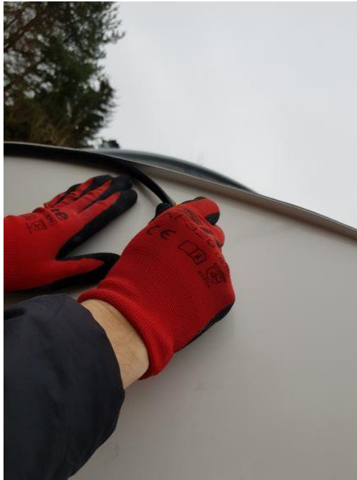
Figure. 68 – mounting the seal on edge of shutter #2
