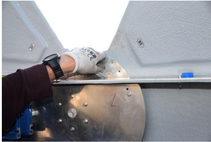
Figure. 49 – Inner washer for shutter No. 2
