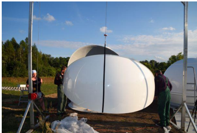
Figure. 47 – shutter No2 transport to top of base
