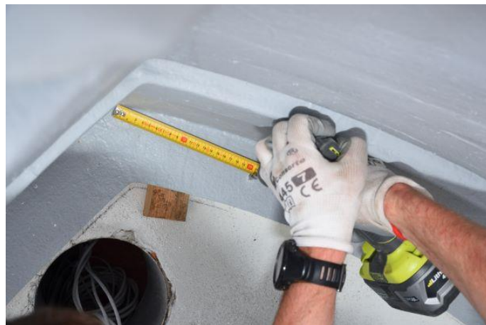
Figure. 12 – drilling of base fixing holes
