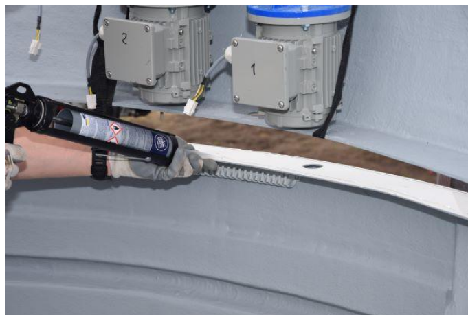
Figure. 20 – sealing of the observatory base elements
