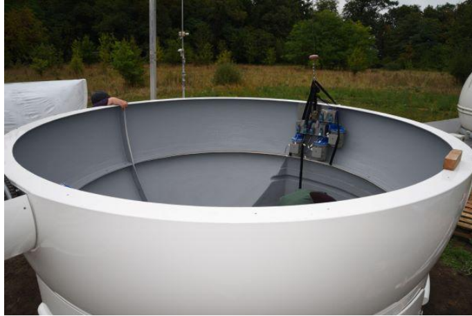
Figure. 24 – Place of sealing of the upper elements of the observatory base
