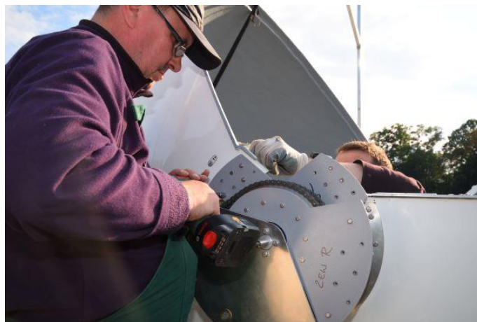
Figure. 42 – screwing the shutter #1 to its mounting handle
