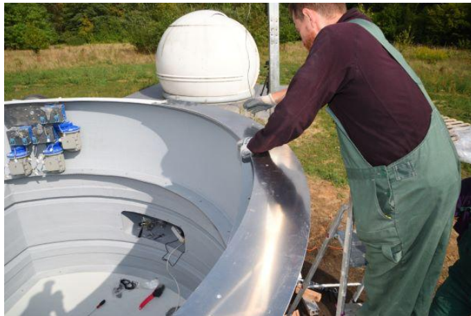
Figure. 29 – Securing the ring with mounting screws
