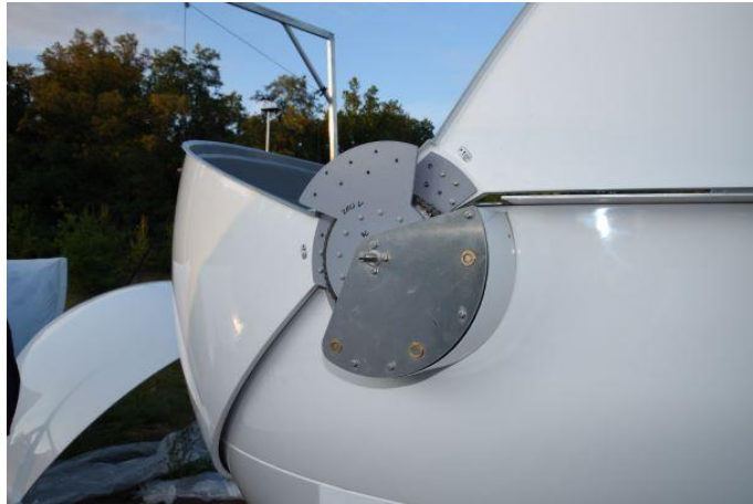
Figure. 49 - Shutter #2 in a partially open position. Shutter No. 1 in closed position.
