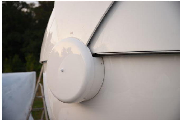
Figure. 61 – Mounted drive unit cover – left side, view at the front of the observatory.
