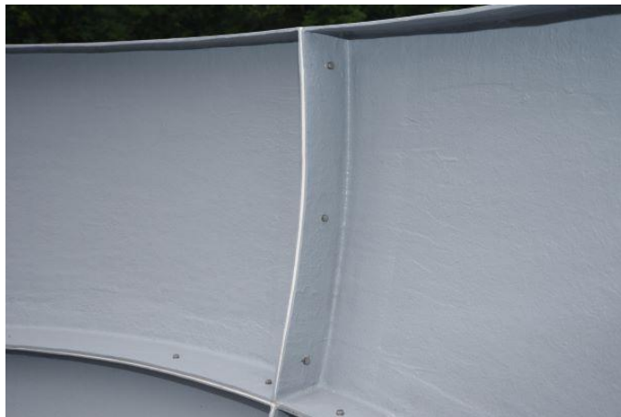
Figure. 25 – Screw connections of the upper elements of the observatory base
