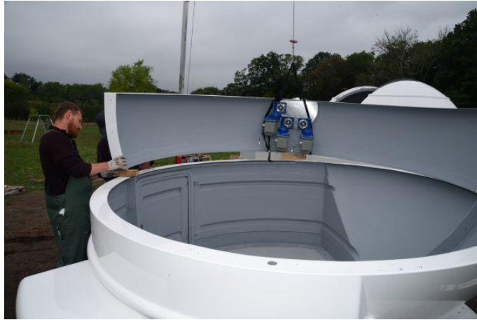
Figure. 19 – preparation for installation of the top of the observatory base
