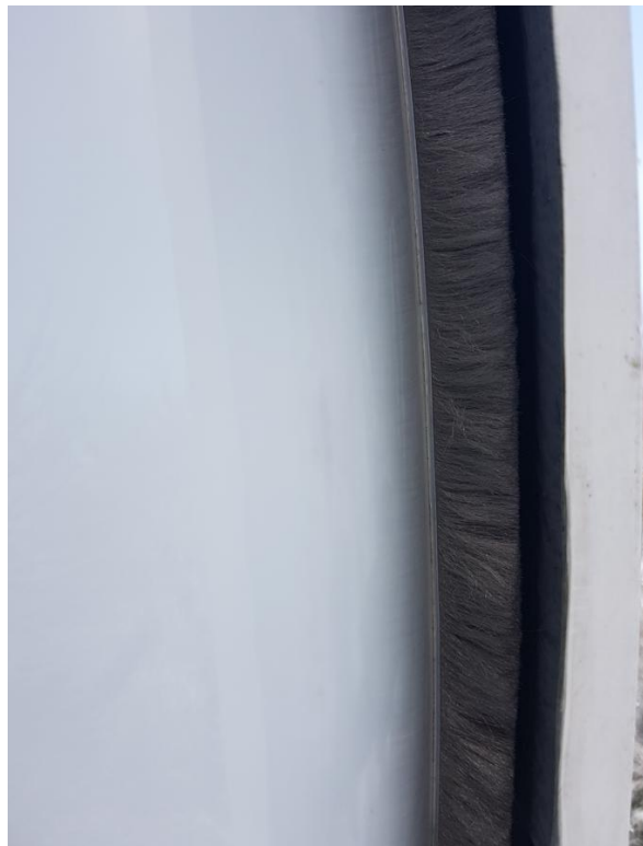
Figure. 69 – Placement of the seal on back edge of shutter #1
