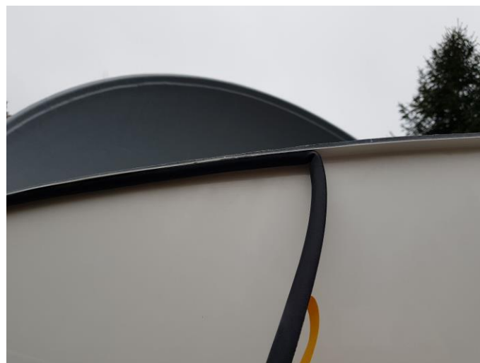
Figure. 67 – mounting the seal on shutter #2
