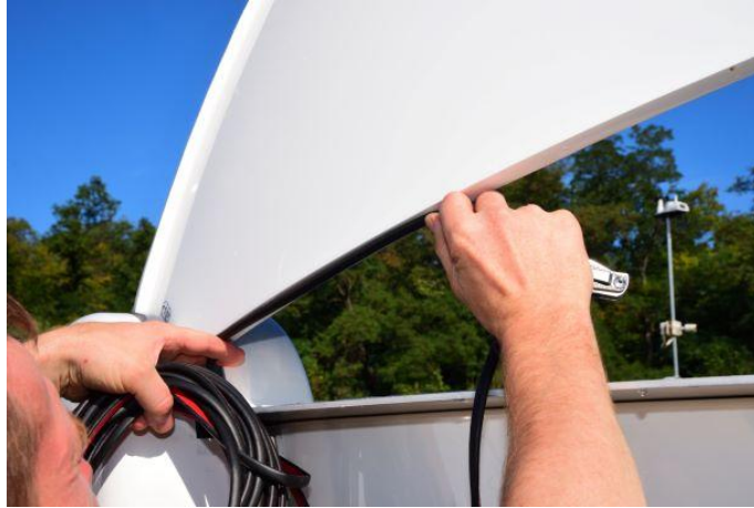
Figure. 63 – Opened shutter #1 for the installation of the seal.
