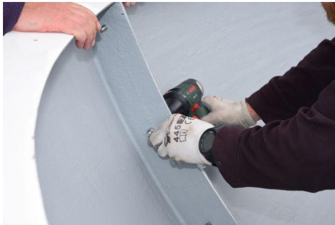
Figure. 18 – connecting the bases of the observatory with screws
