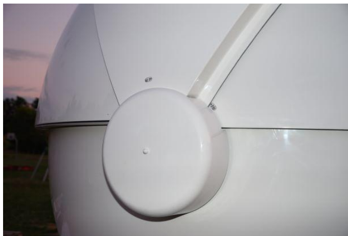
Figure. 62 – Mounted drive unit cover – right side, rear view of the observatory.
