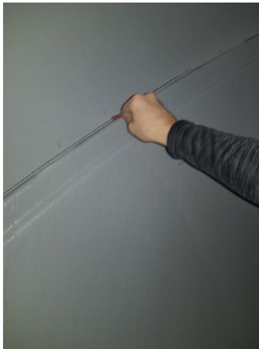
Figure. 69 – Marking the line for mounting a seal on shutter #3
