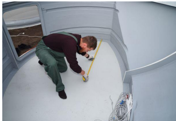
Figure. 9 – measurement of observatory position relative to the centre of the slab
