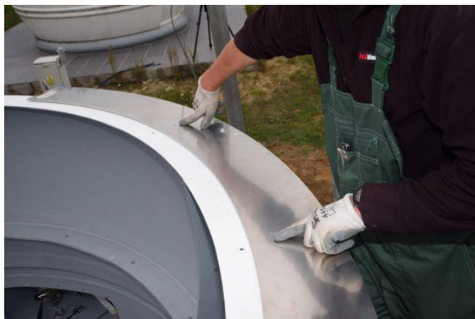
Figure. 27 – Ring fixing holes to the base of the observatory
