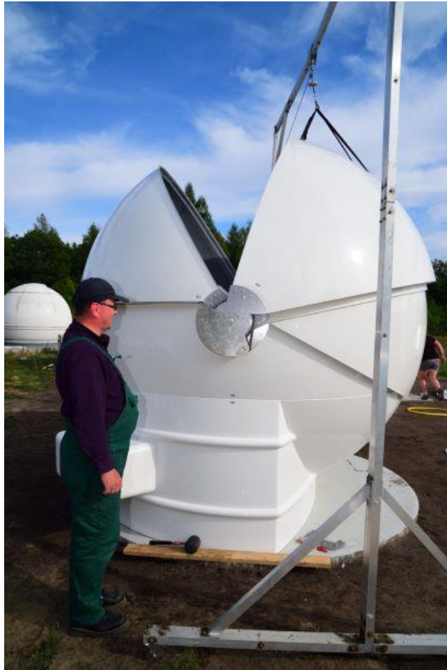
Figure. 54 – mounted shutter No. 3 mounting in its handles
