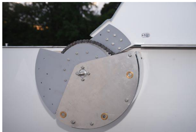
Figure. 43 – Screw connections of shutter #1 upon its mounting handle
