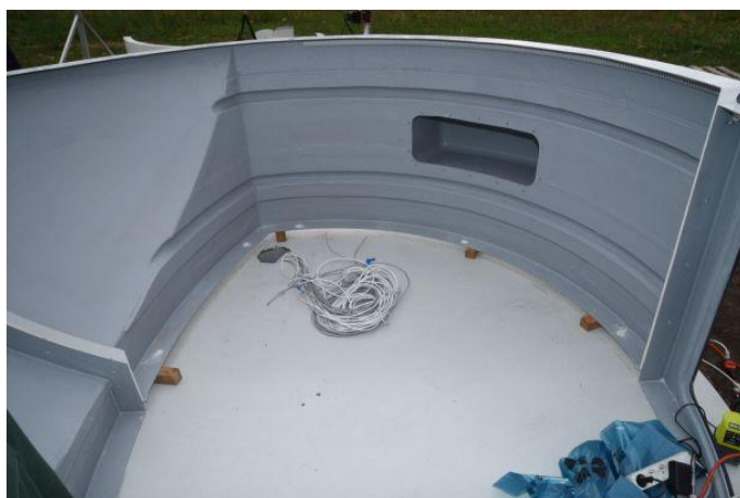
Figure. 13 – drilled holes in one of the bases of the observatory
